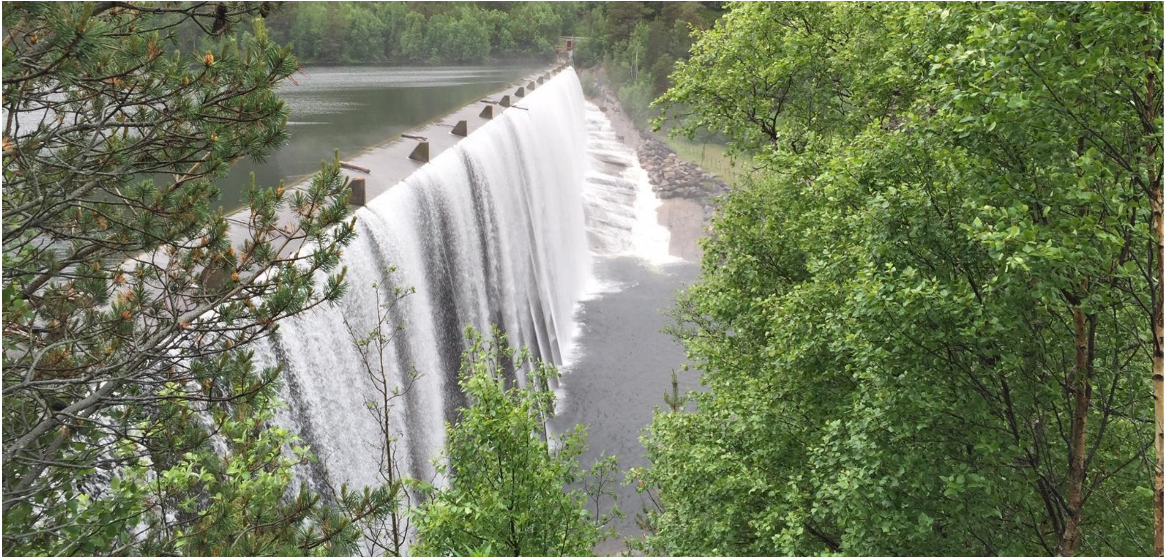
Litjfosse dam, Orkla sub-district ©Bendik Eithun Halgunset
