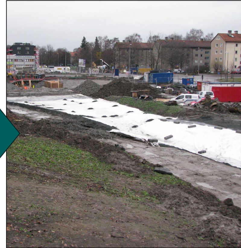
Construction Phase in 2014. Photo: Anders Iversen.
