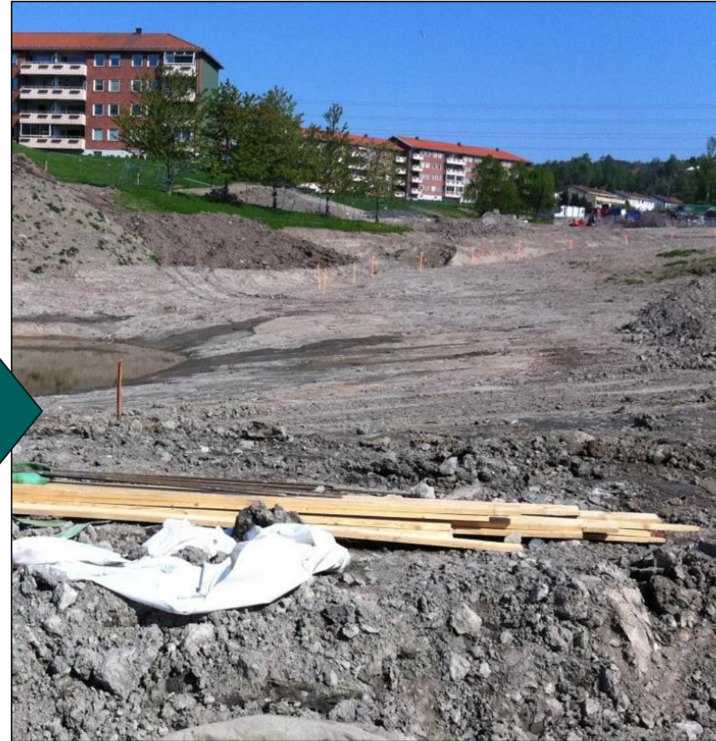
Construction Phase in 2013. Source: Oslo Municipality.
