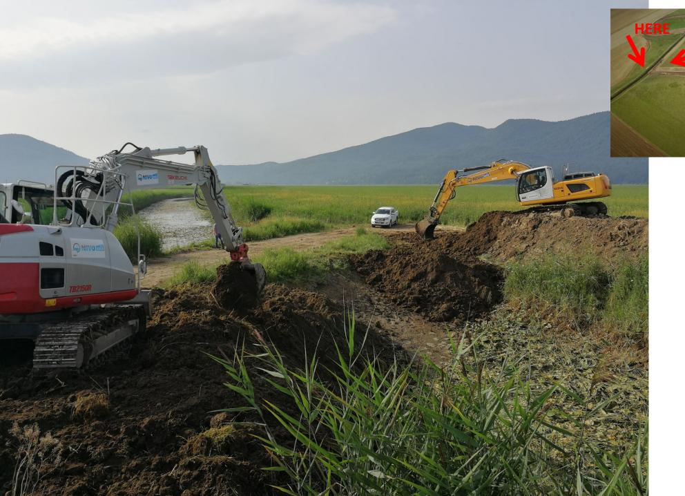
Then, we started putting soil in the dry canal, starting from the upper part and working from both sides of the channel.
