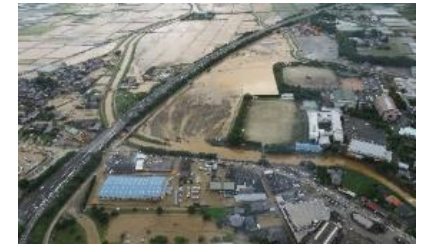
④ Inundation (The Katsura River) (Asakura-city, Fukuoka)
