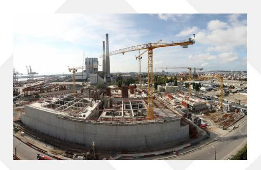
Demolition of the existing treatment plant of Le Havre dating from 1968 and construction of a new station which fulfills, in particular, the European requirements relating to the treatment of nitrogen and phosphorus.
