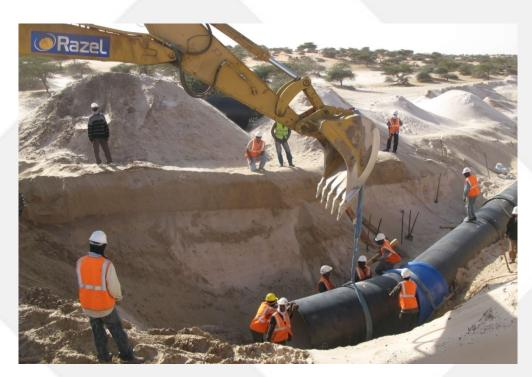
As part of the market of water transfer from the Senegal River to supply water to Nouakchott, RAZEL performs all work in the trenches, tracks and platforms. The design of the project was expected to produce 170 000 m³ of water per day to meet demand until 2020. Arrangements were already planned to bring production to 226 000 m³ per day.
