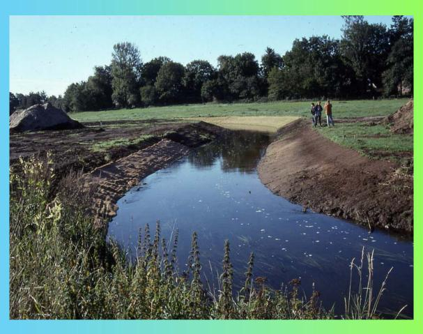
Limit morphological reconstruction to cases with low natural recovery potential (low-energy, low sediment load channels) or constrained (urban channels)
